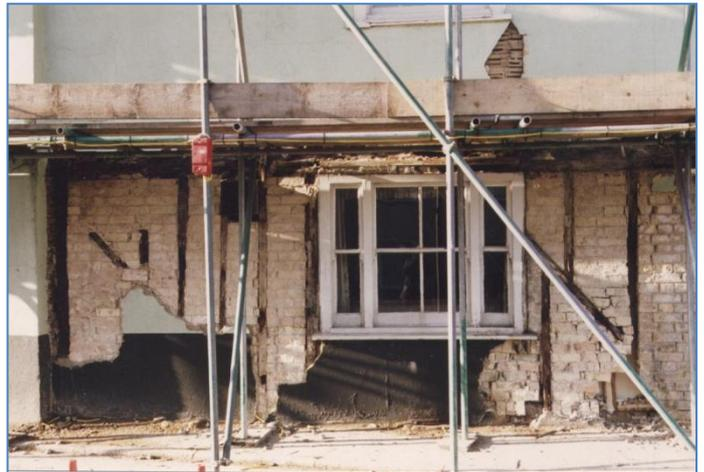
Enlargement of the front wall showing laths, timbers and brickwork (1992)
